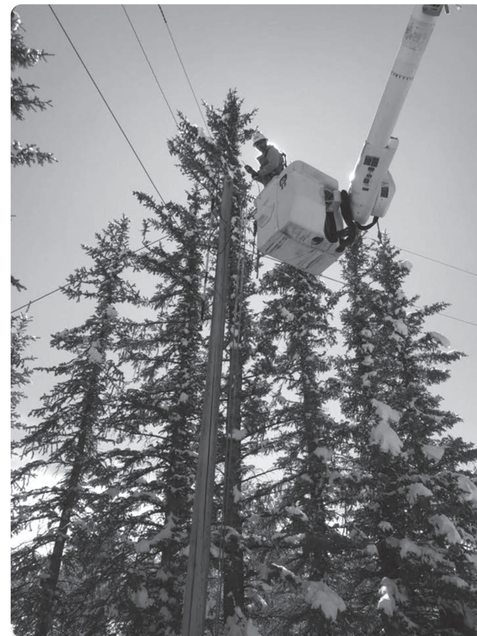
JOURNEYMAN LINEMAN TRAPPER BRADSHAW REPAIRING DOWNED LINES
