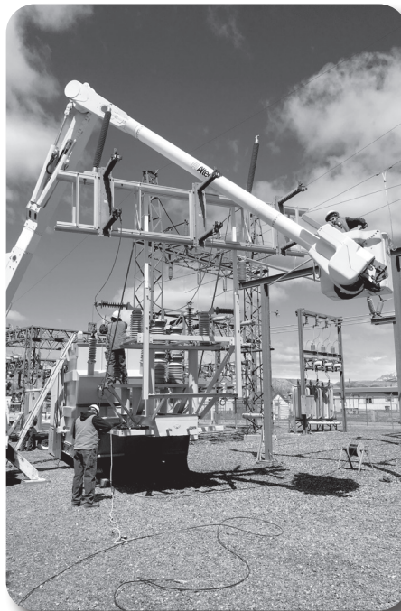
A 10-megavolt amp (MVA) transformer was purchased and replaced an existing 5 MVA transformer at the Henthorne sub.
