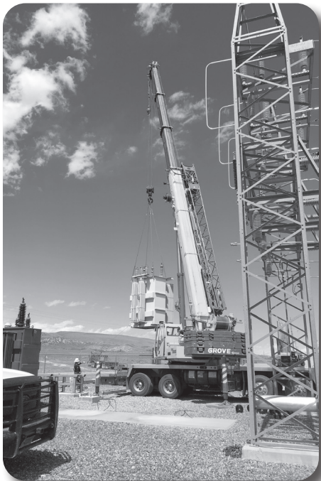
A 10-megavolt amp (MVA) transformer was purchased and replaced an existing 5 MVA transformer at the Henthorne sub.
