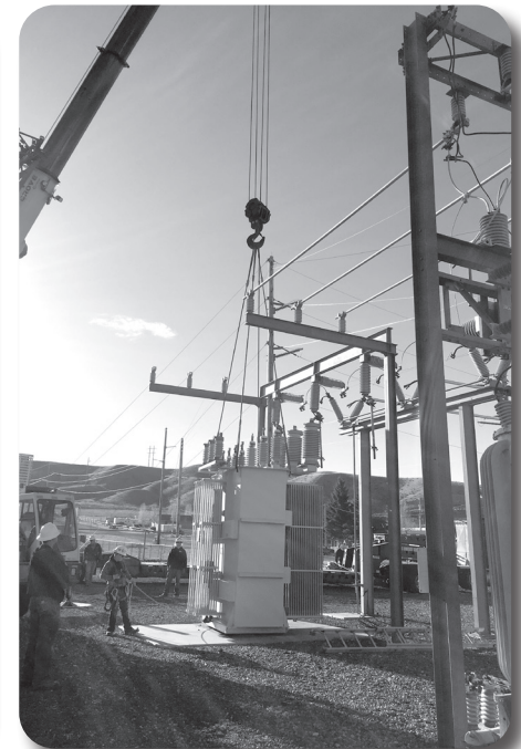
A 10-megavolt amp (MVA) transformer was purchased and replaced an existing 5 MVA transformer at the Henthorne sub.
